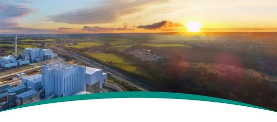
enfinium is proposing to install carbon capture and storage (CCS) technology at its Ferrybridge 1 and 2 facilities in Knottingley, West Yorkshire. Installing CCS at these two facilities would capture around 1.3 million tonnes of carbon dioxide ( $CO_2$ ) each year by the time both facilities are operational.
